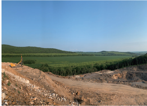
Figure 8–11: The planned beneficiation plant at Beishan, looking to the southeast
