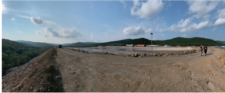
Figure 8–7: Current tailings storage facility, looking from the southeast to northwest
